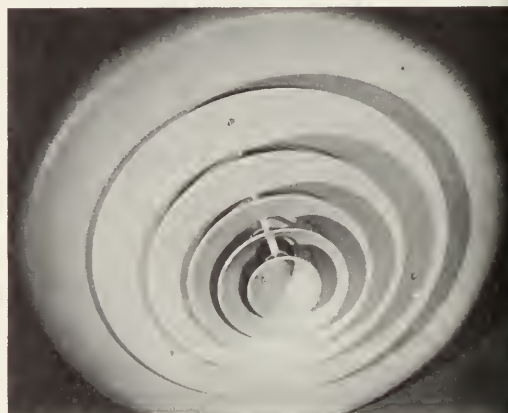
23-5. A ceiling grille that diffuses the air as well as it delivers it to the room. (Anemostat Corp. of America)
